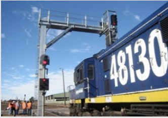
MGB Provides integrated Signalling services from concept design through detailed design including testing and commissioning
